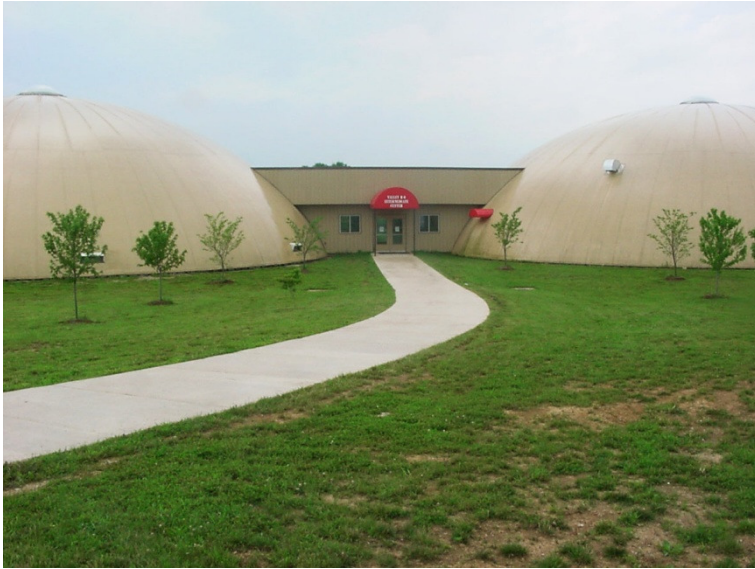
Two of the five monolithic domes at Valley R-6 Elementary School
