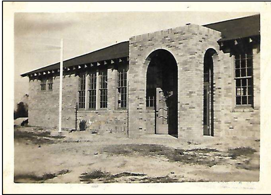
West side of new school building—Main entrance with flag pole
