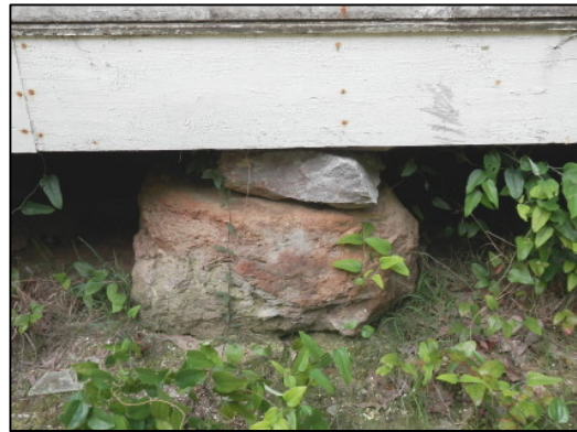
Foundation stones at Carolina Church
